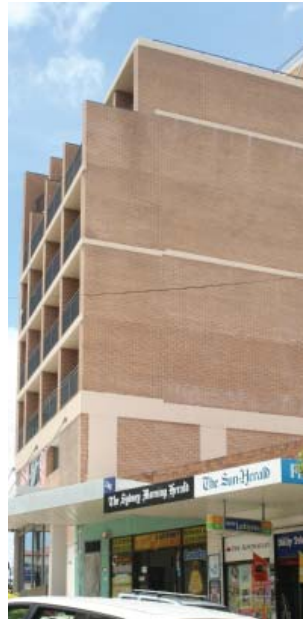
Example of blank facade of a taller building seen behind a lower level development.
